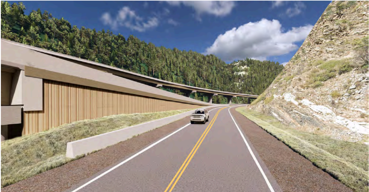
Wall Treatment: 5x10 panels
