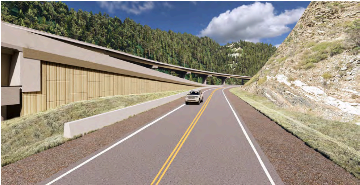
Wall Treatment: 5x5 panels
